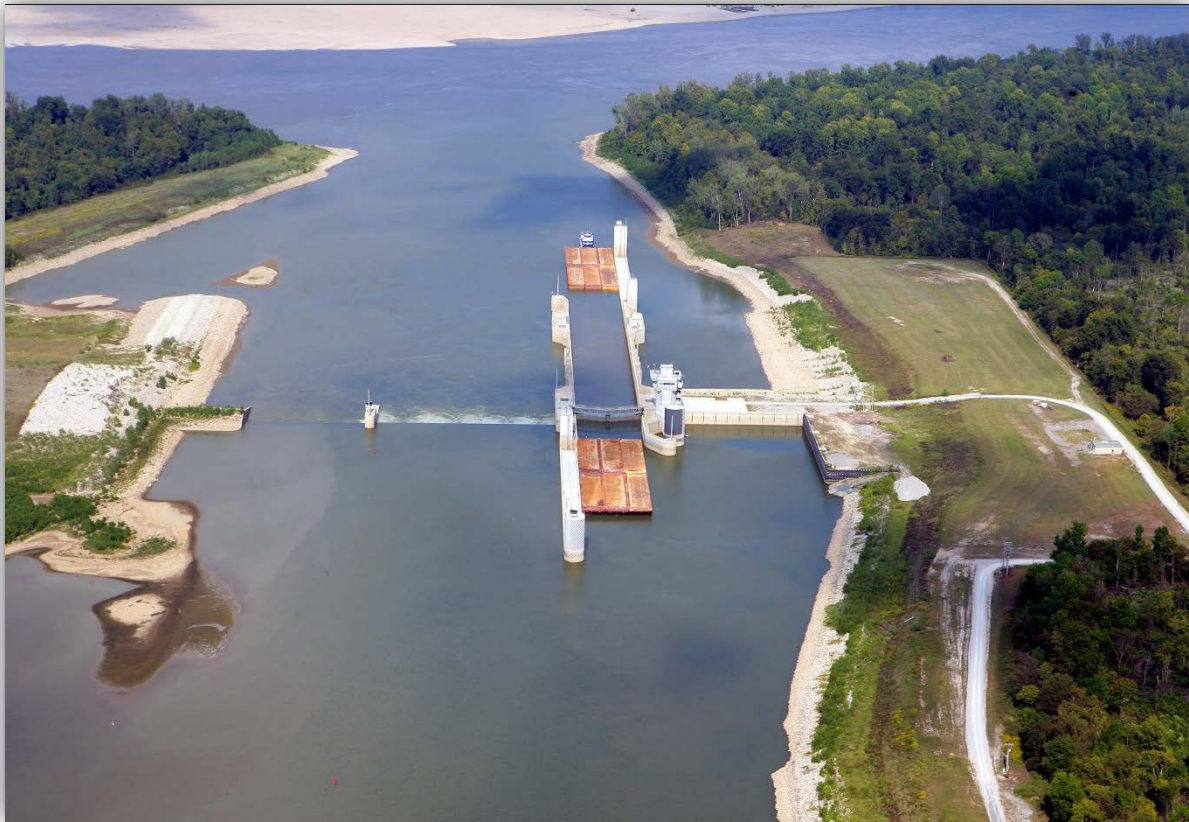
Photograph: Entrance channel to the McClellan Kerr Arkansas River Navigation System and Montgomery Point Lock and Dam at the confluence of the Mississippi and White rivers, Arkansas
